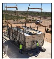
A filter unit is placed on a concrete pad awaiting installation of ducting.
